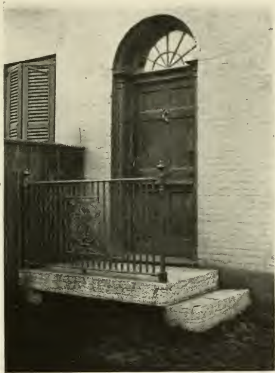
One of the Entrances to the Residence of Hon. A. A. Yates, on Washington Avenue.
